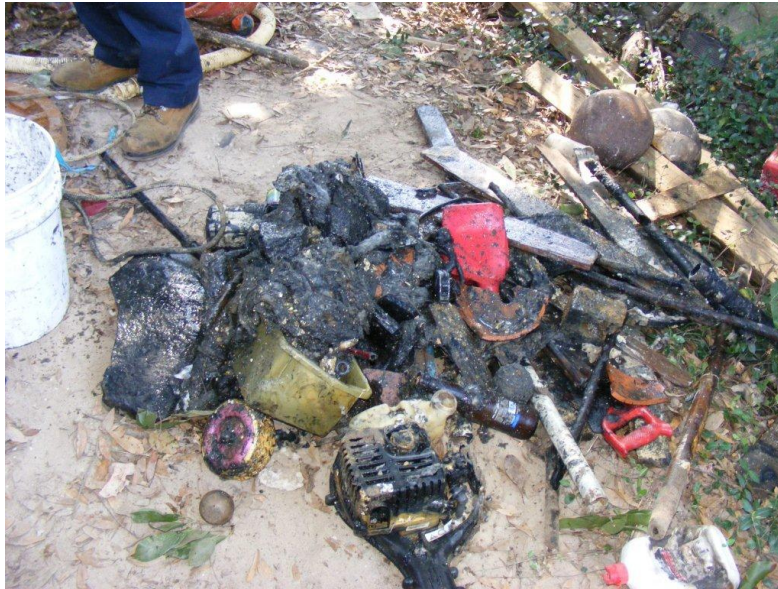
MAWSS crews removed assorted debris from manhole near Bridgewood Ct.
