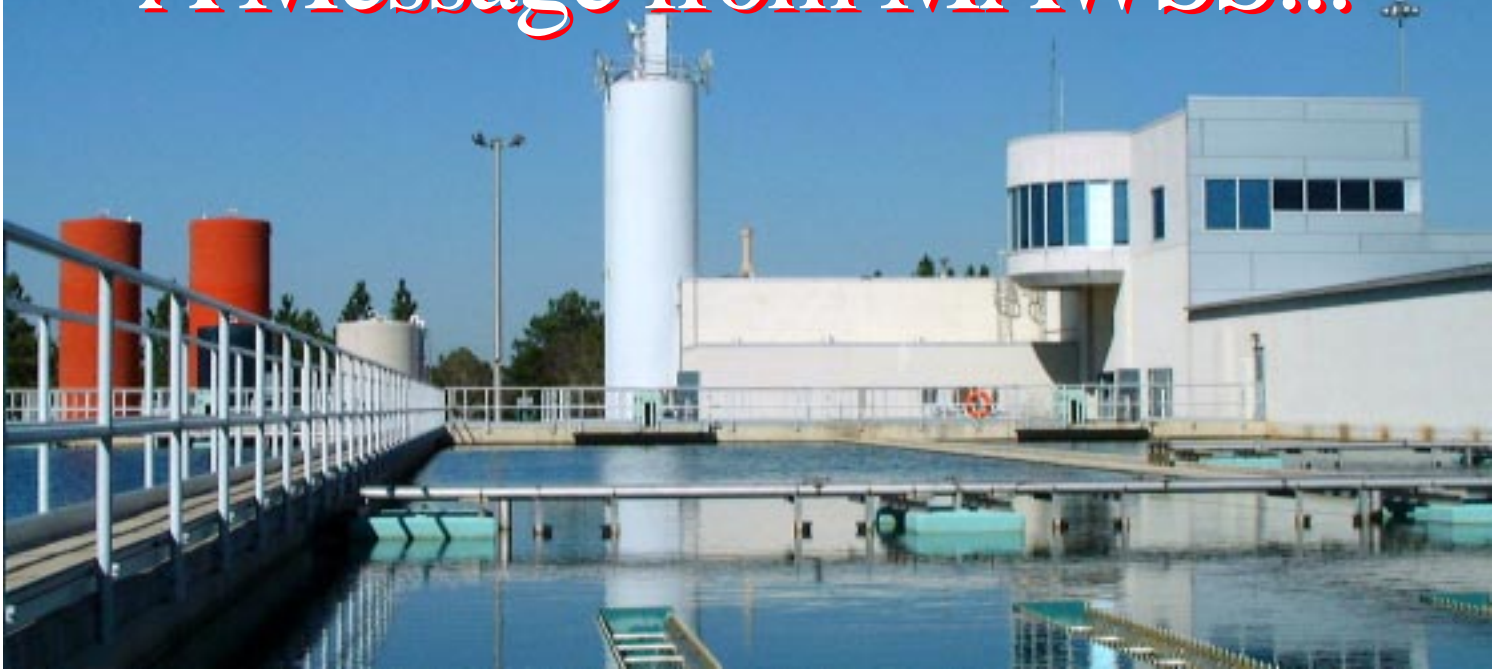
The Myers Plant is one of two water filtration facilities that process the water from Converse Reservoir for distribution to MAWSS' 300,000 customers.
