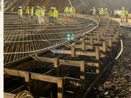
Cover Photo: Construction of severe weather attenuation tanks (SWATs) in Mobile is expected to be completed by December 31, 2020. There are two new SWATs adjacent to an existing tank near Tricentennial Park. SWATs provide temporary storage during heavy rain events.
