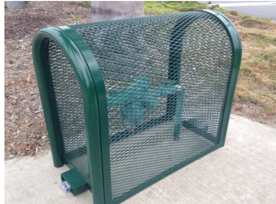
Residential Backflow Prevention Assembly with Locked Enclosure
