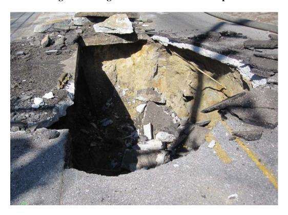
Crews from Mobile Area Water & Sewer System (MAWSS) are repairing an 18-inch sewer line on Sage Ave. causing traffic to be rerouted between Old Shell Rd. and Dauphin St. MAWSS crews discovered a problem during routine cleaning and maintenance of the sewer main that prompted the emergency repair. A video camera used to view the sewer line saw water and soil entering the line, indicating a break. Crews found a large void under the concrete when they opened the road for repairs.
